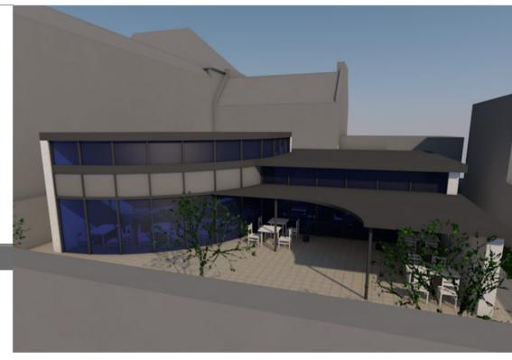
grey membrane flat roof white rendered walls dark grey aluminium faced timber composite windows & screens
