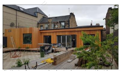
Fig 13 - view from rear garden showing the upstairs residential flat with a chimney stack on its gable elevation through which the kitchen flue will extract
