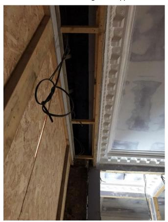
Figure 6 Unsealed gaps at the edge of the separating floor (from within the restaurant)
